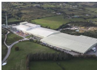
Plant in Derrylin, Northern Ireland.
