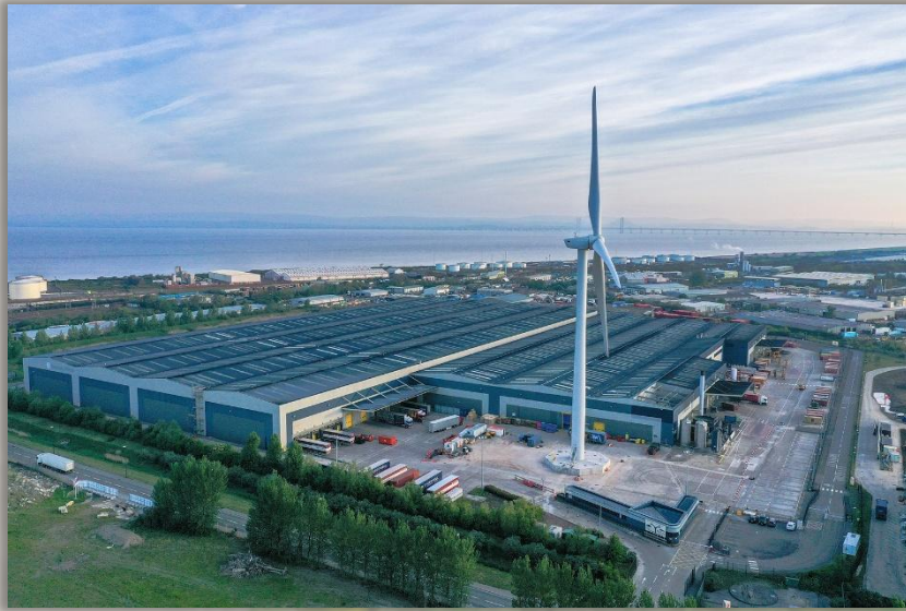
Beverage filling facilities in Bristol, UK.
