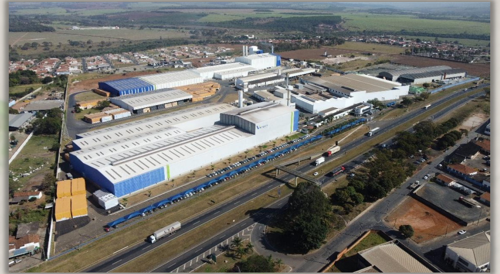
Glass manufacturing facilities in Porto Ferreira, Brazil.
